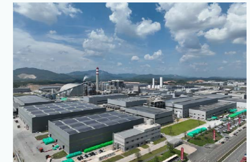
Guangxi base "Source, Grid, Load and Storage" integration project
