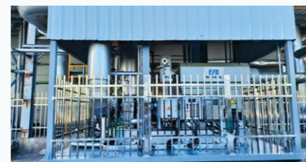
Deploying energy efficiency enhancement equipment
