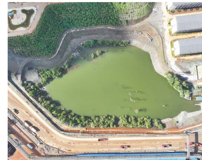
Huafei Company rainwater storage pond
